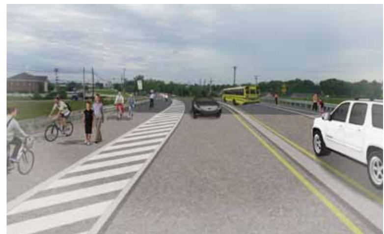
**Conceptual Improvements Across the Existing U.S. 27 Bridge.** The U.S. 27 bypass bridge that crosses KY 29 would be widened 18 feet to provide a sidewalk and path with a raised buffer to protect people from the passing cars as illustrated here.
